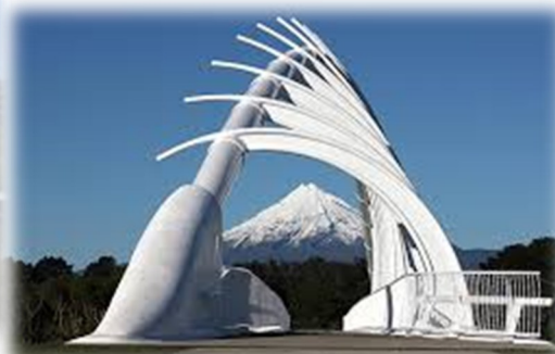
Te Rewa Rewa Bridge
