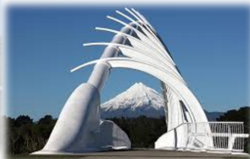
Te Rewa Rewa Bridge
