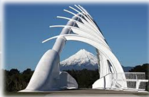
Te Rewa Rewa Bridge
